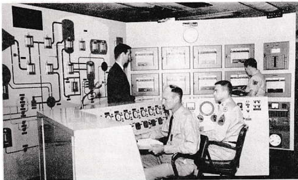
Control Room. This is the nerve center of operation at the SM-1. From this room the reactor is controlled by manipulation of the control and safety rods. The various meters, indicators and recorders, shown in the photo, are indicating or recording various plant parameters.
